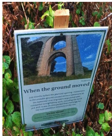
third arch had to be shored up because of subsidence
