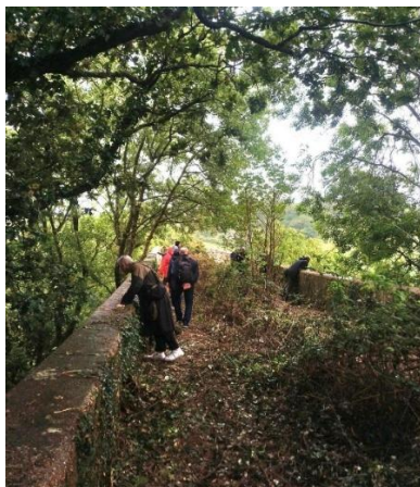
Walking across the top of the Viaduct
