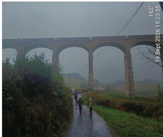
Cannington viaduct in the rain
